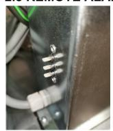
These units are equipped with remote alarm terminals for the connection to a remote alarm network.
